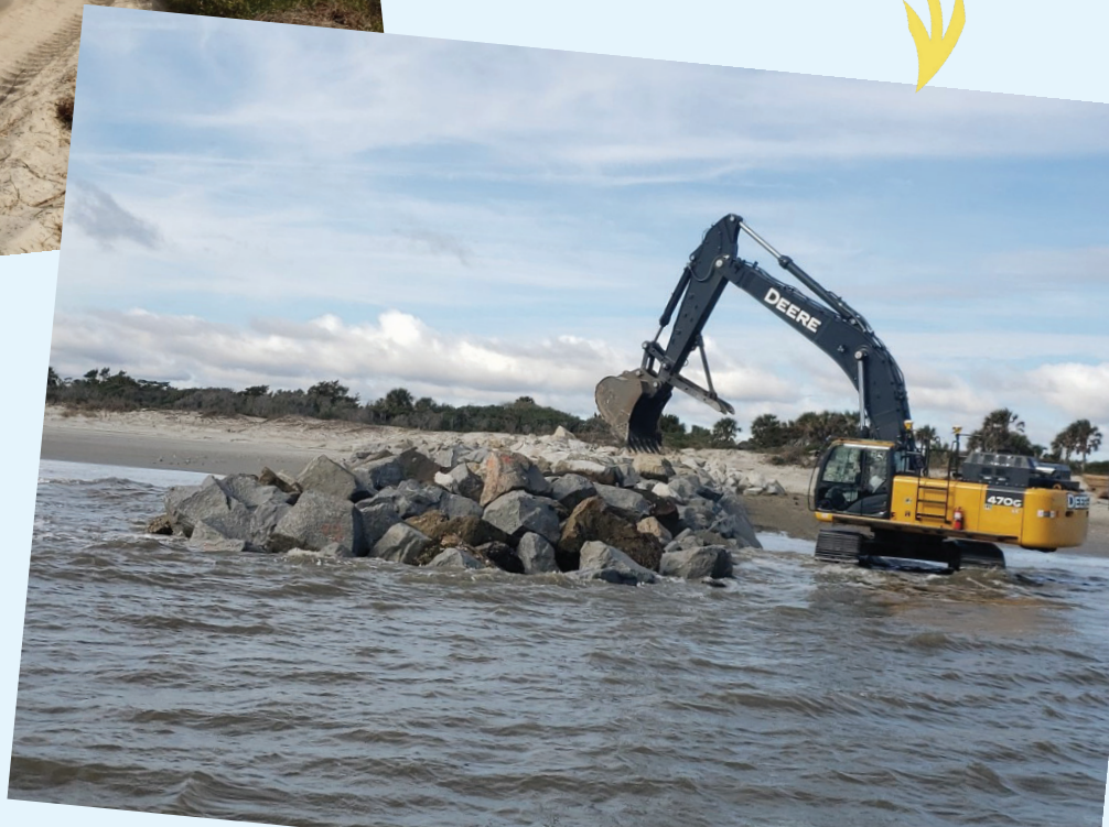
Backhoe places rocks onto jetty structure
